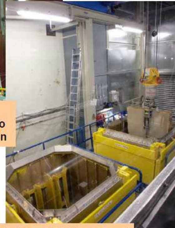
Packing of RPV segment into KONRAD container
