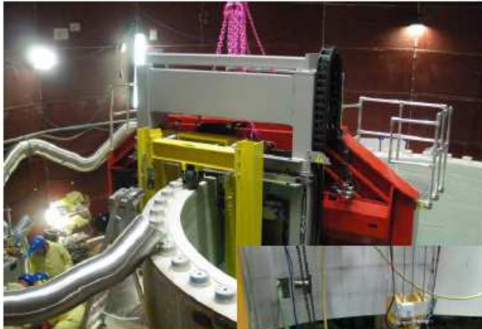
Vertical segmentation of RPV flange
