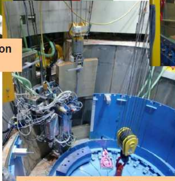
Gripper removing RPV segment
